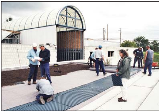
Installing the green roof layers at GreenForge.
