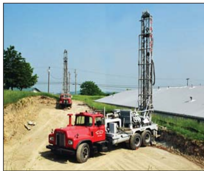
Drilling geothermal wells at GreenForge
