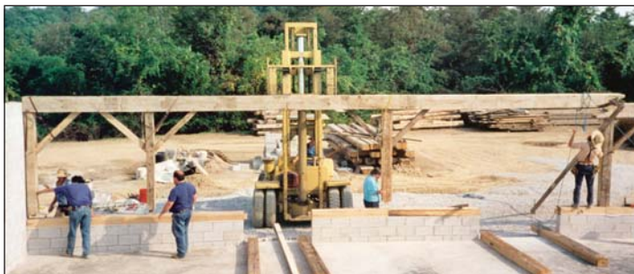
Raising the 125-year-old barn timbers at their new location.
